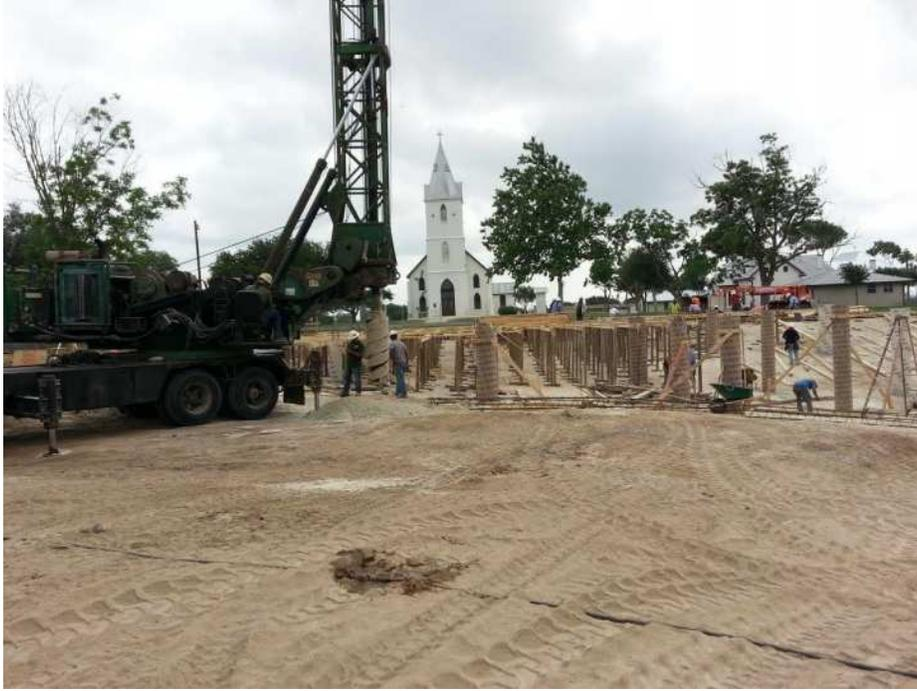
Continuation of drilling of the piers and the construction of the form for the foundation, Week 5
