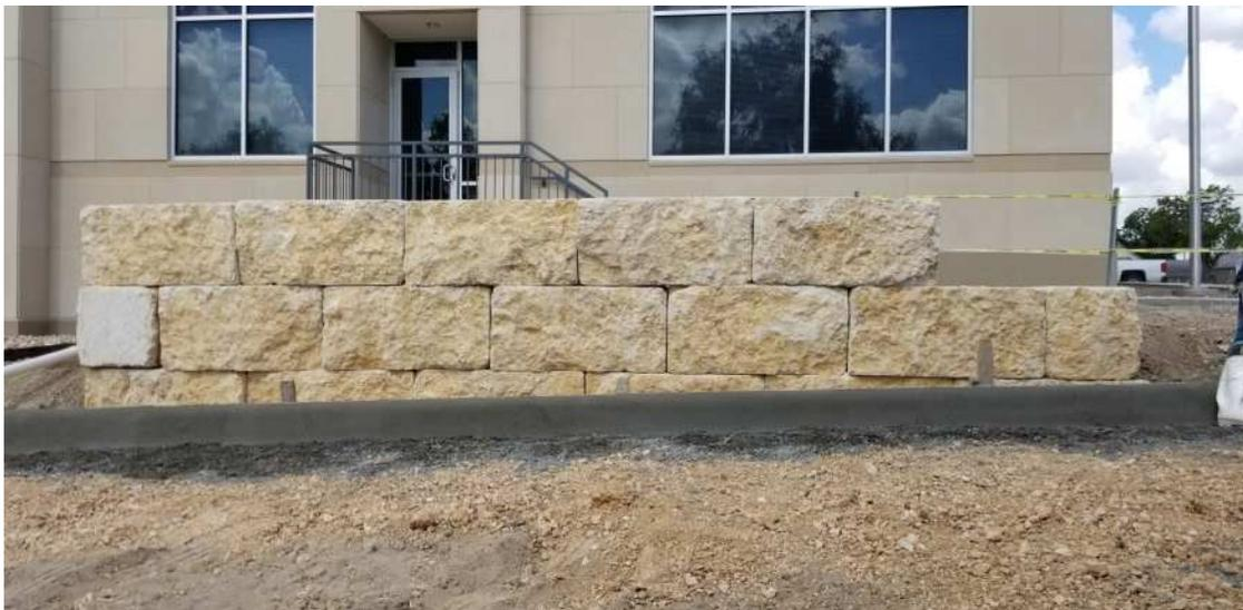
Large limestone blocks installed on the south side and the inner curb is poured.
